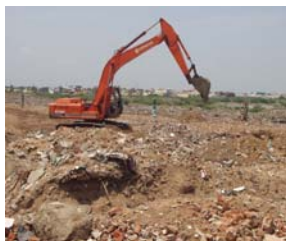
Leveling at Dumpsite
